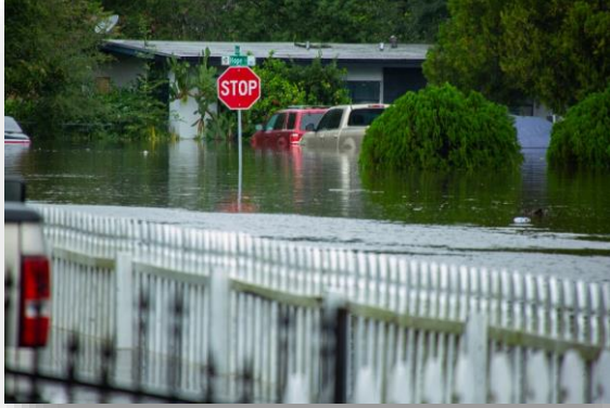
Figure 4. Hurricane Ian Impact on Residential Neighborhoods Source: Orange County Government, October 2022
